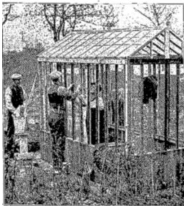
Figure 29. Men at the Warriston site constructing a greenhouse from old photographic plates. ( The Scotsman January 1935)
