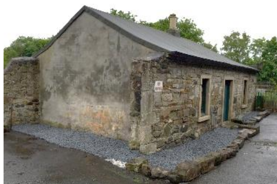
Figure 40. Cottage with stone chippings laid. 2015. (Photo by Rik Hart)
